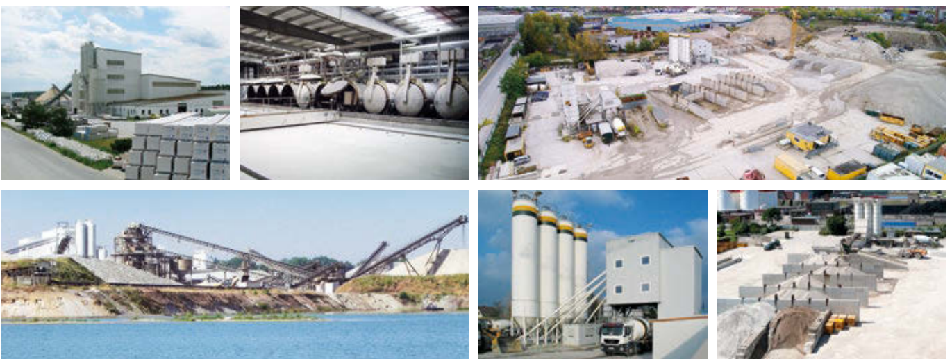
LÖBNITZ GRAVEL/BUILDING MATERIALS PLANT
