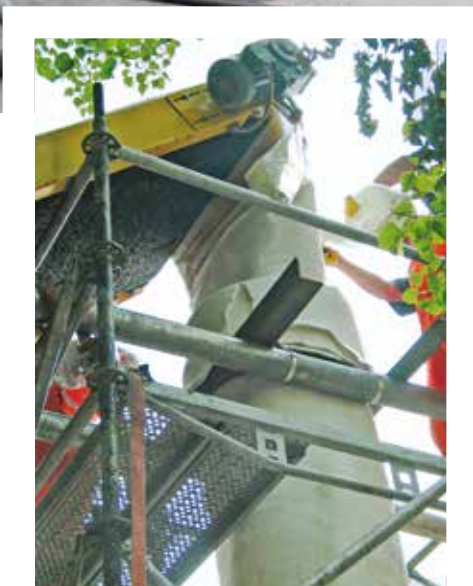
The in-liner is inserted into the reach via the inversion tower
