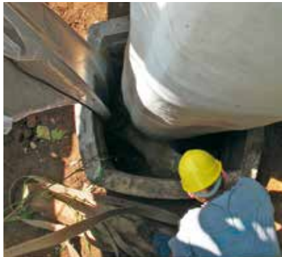
Insertion of the hose liner into the egg-shaped section
