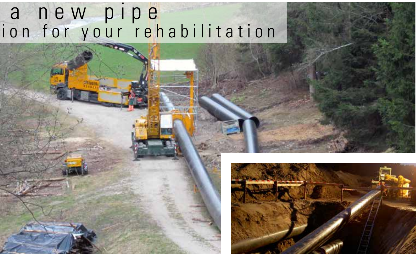
DynTec rig and pipe run
