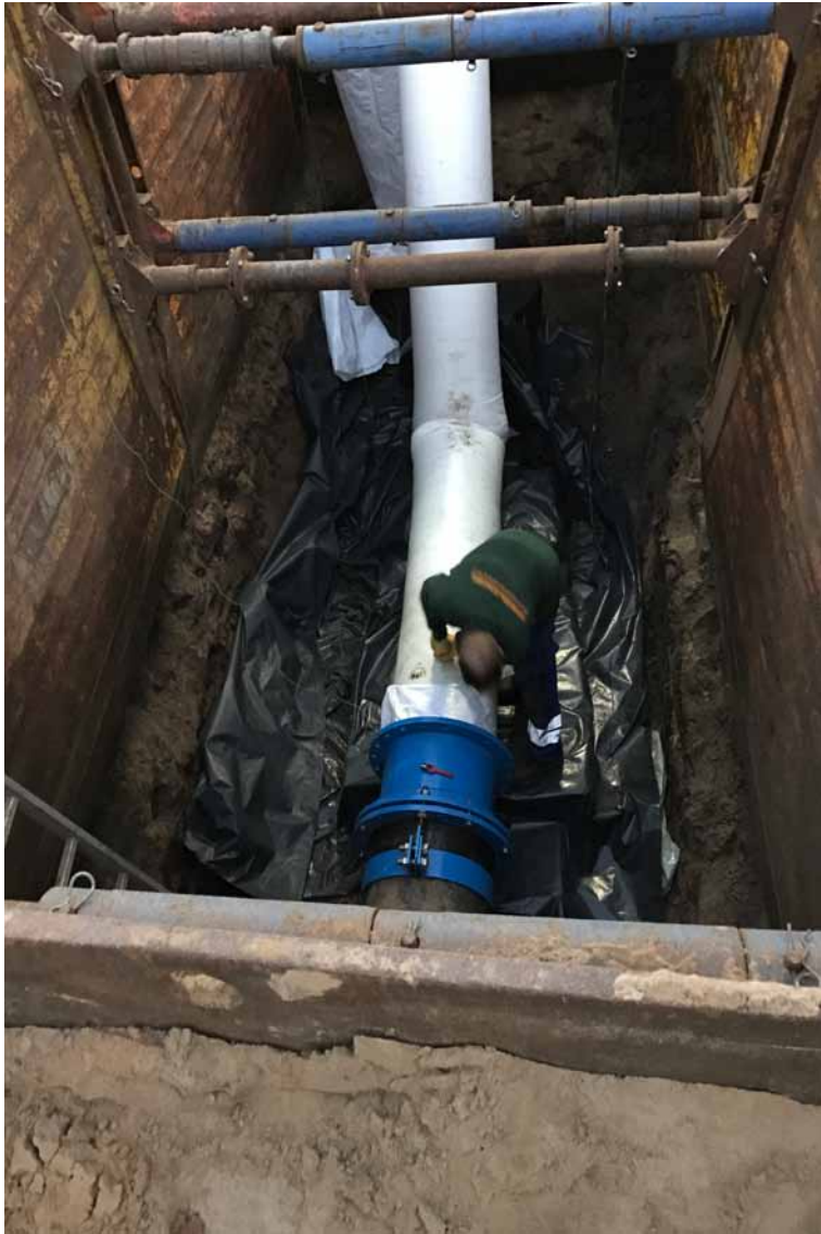
Installation des BlueLiners.
